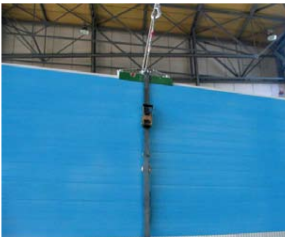
Pic. 8. Using lifting assembly tool with sandwich panels in horizontal panel arrangement.
